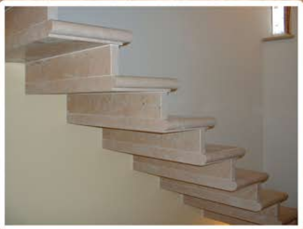
SELF LOAD-BEARING STAIRS IN PINK BRUSHED LESSINIA STONE THICKNESS OF 6 CM
