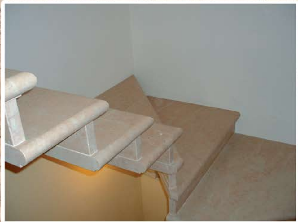
SELF LOAD-BEARING STAIRS IN PINK BRUSHED LESSINIA STONE THICKNESS OF 6 CM
